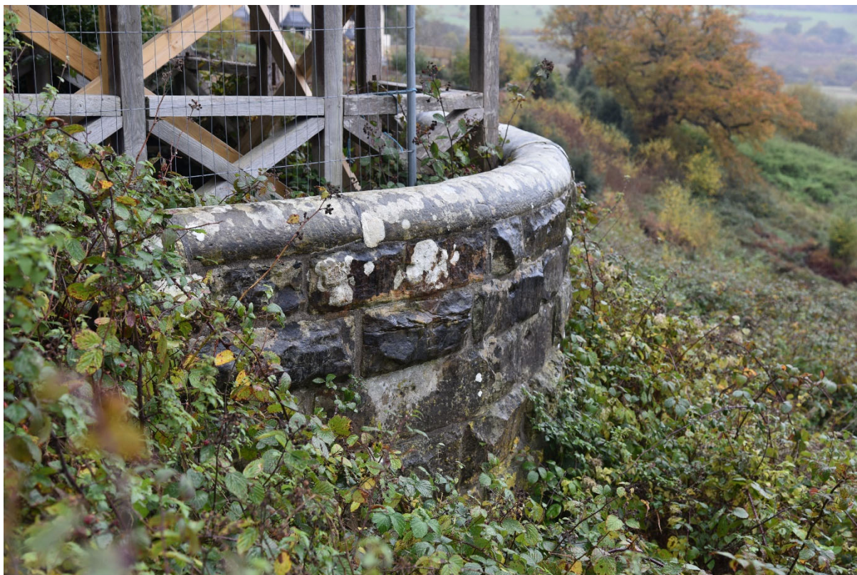
Plate 13: Detail of the perimeter wall.
