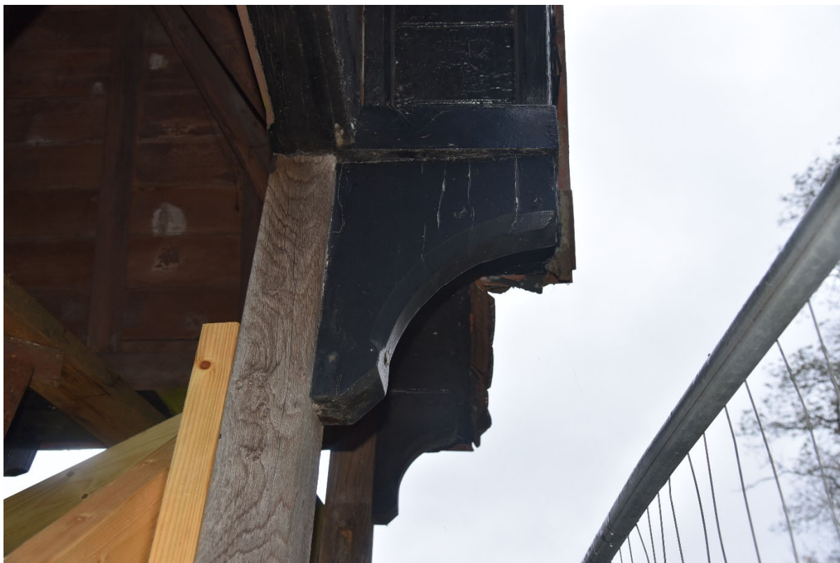
Plate 9: Detail of carved eaves brackets.
