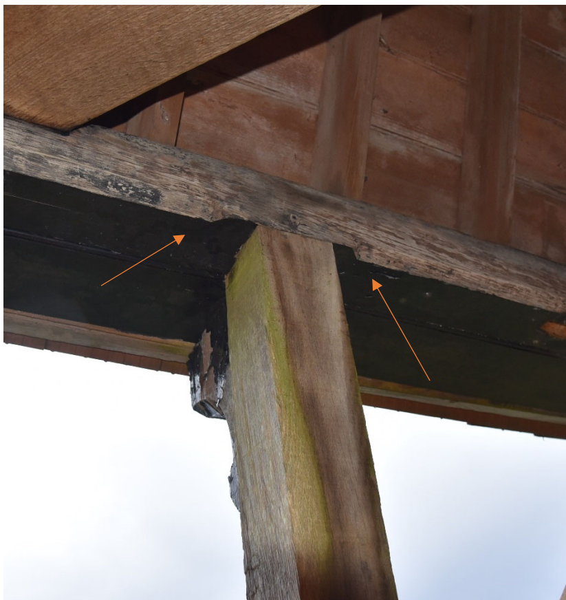
Plate 5: Detail of chamfer-stops to wallplate (highlighted).
