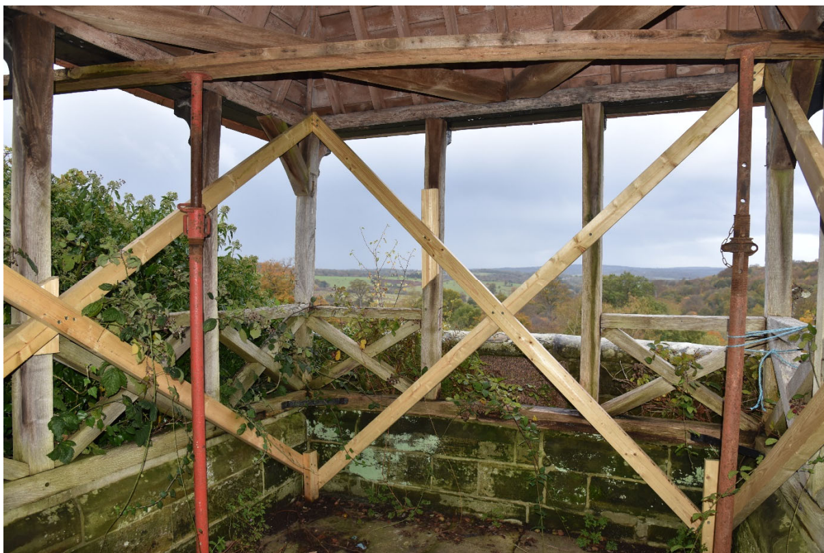
Plate 2: The interior of the building, looking south-west.
