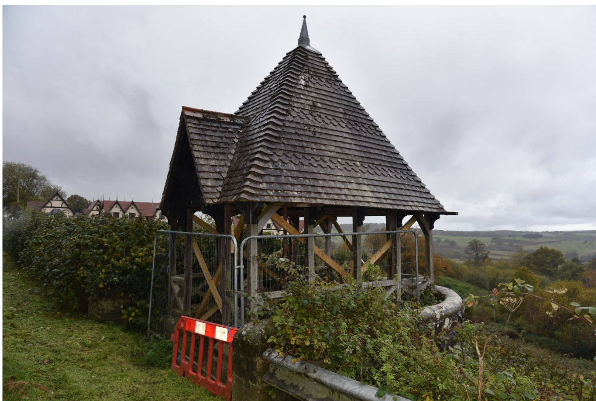
Plate 12: Looking south-west, showing the well building set within the perimeter wall.
