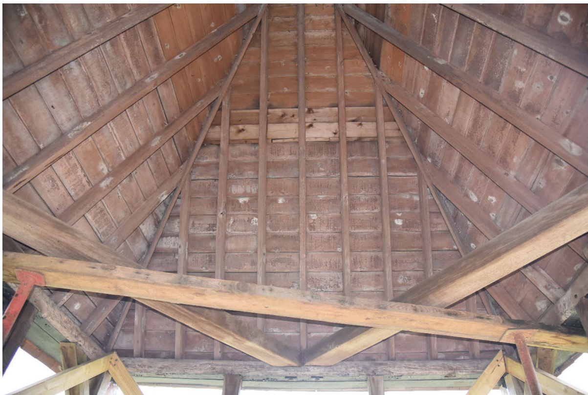
Plate 7: The roof structure, looking west. Note the dragon ties.
