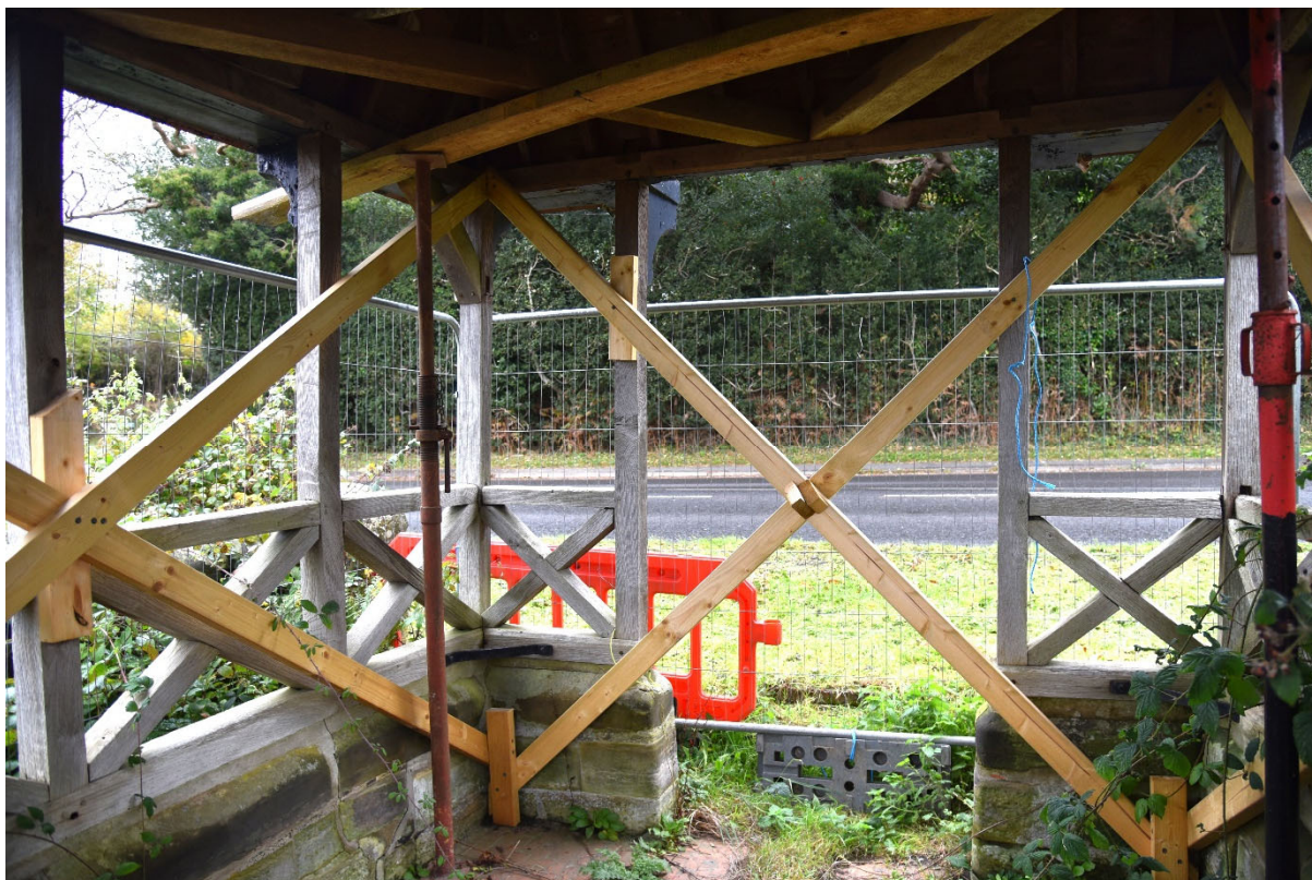
Plate 3: The interior of the building, looking north-east.
