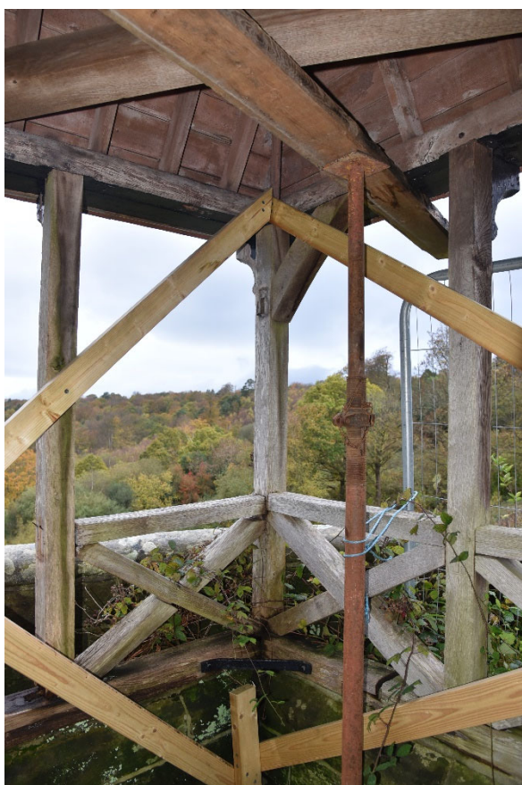
Plate 4: Detail of the framing at the north-west corner.
